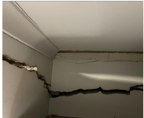
Figure 2: The cracked wall due to subsidence
