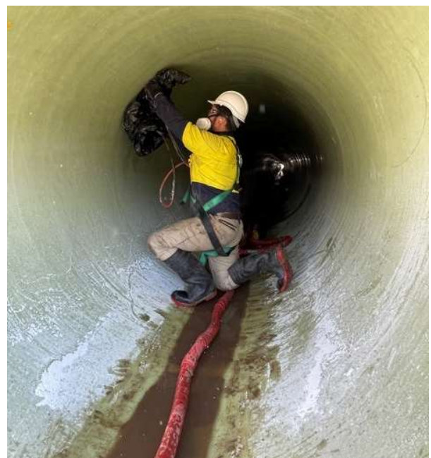
Figure 2. Internal Resin Injection Through New Pipe Lining
