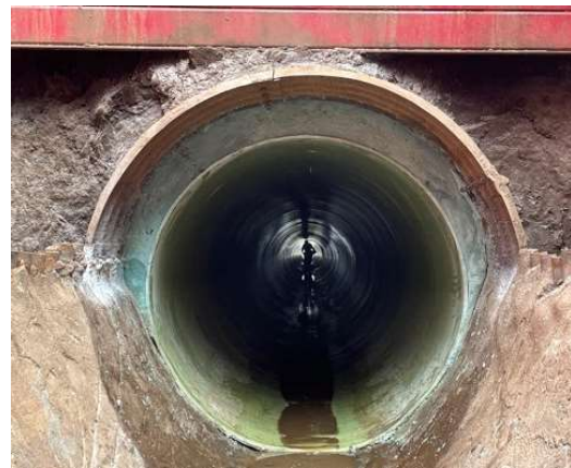
Figure 4. Annulus Filling Completed
