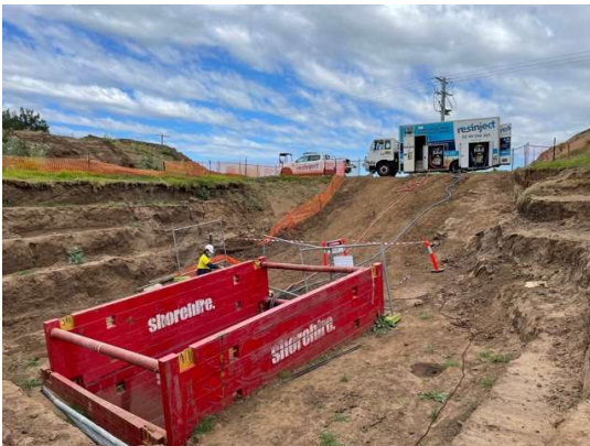
Figure 1. One of the Access Points for the Relined Pipe
