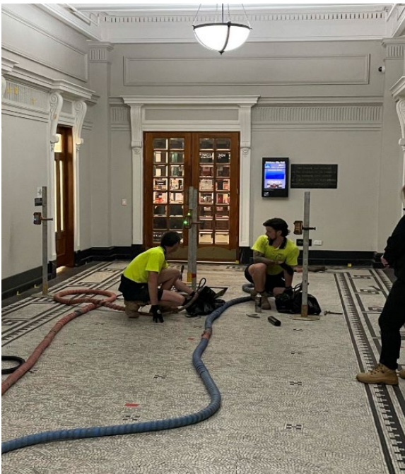
Figure 3. Lobby with Resinject Treatment Underway
