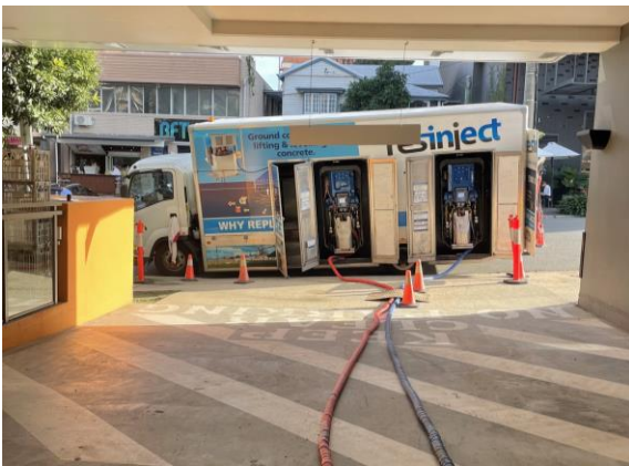
Figure 1: The Resinfect Rig with its two pumps delivering our RSJ170 Resin to the impacted car parks.
